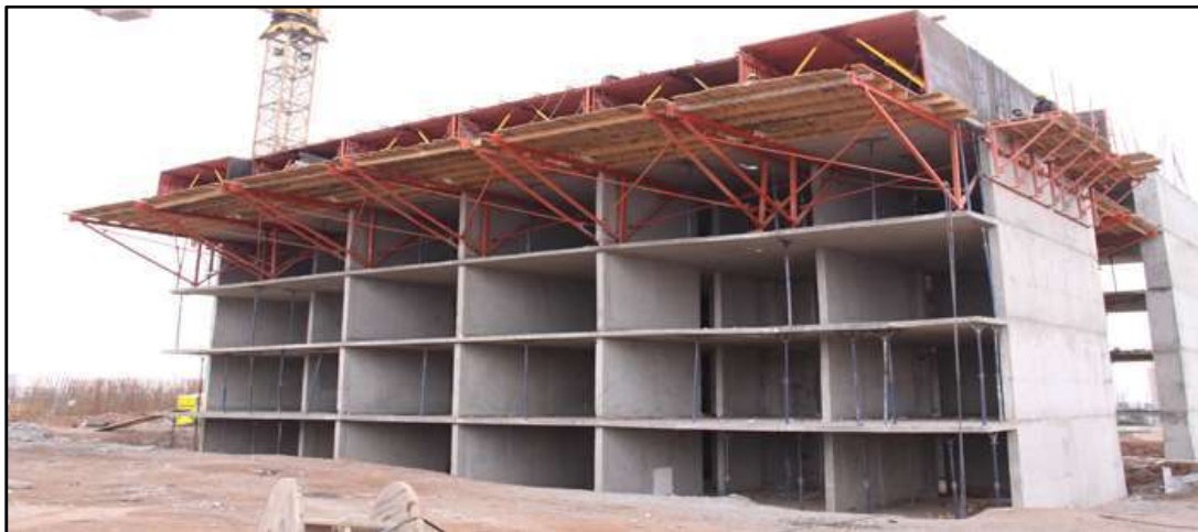
Fig. 87 Tunnel Formwork System
