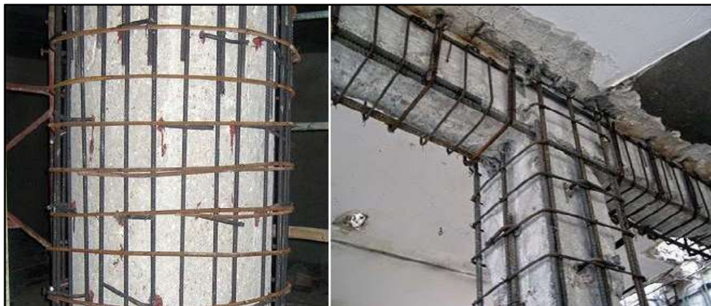
Fig. 84 Jacketing of Column and Beam
