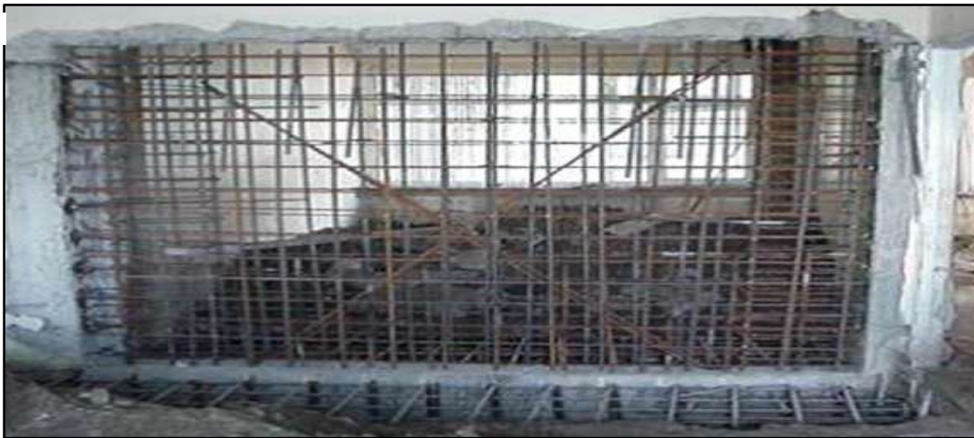
Fig. 82 Adding New Shear Wall
